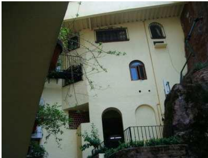
The South Side of the Building was painted recently with the addition of the Ramp to the Lobby.
