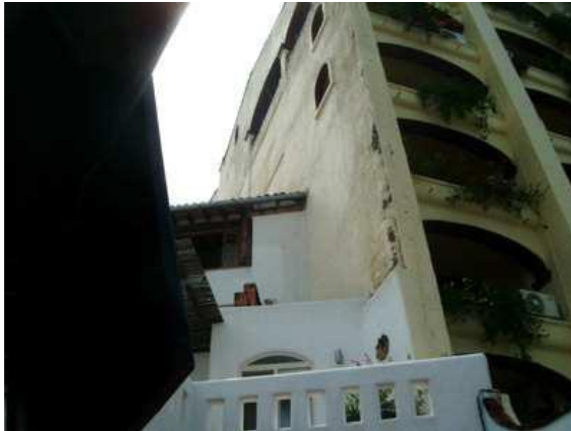
Future Painting of the Building has been included in this Study.
